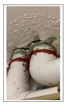
space creating a fire passage point into the plenum, (space between floors) in the building. This open annular space has compromised the fire rated continuity of this room and the building. A fire in this room would easily spread into the plenum through the non-protected annular space and spread through the
