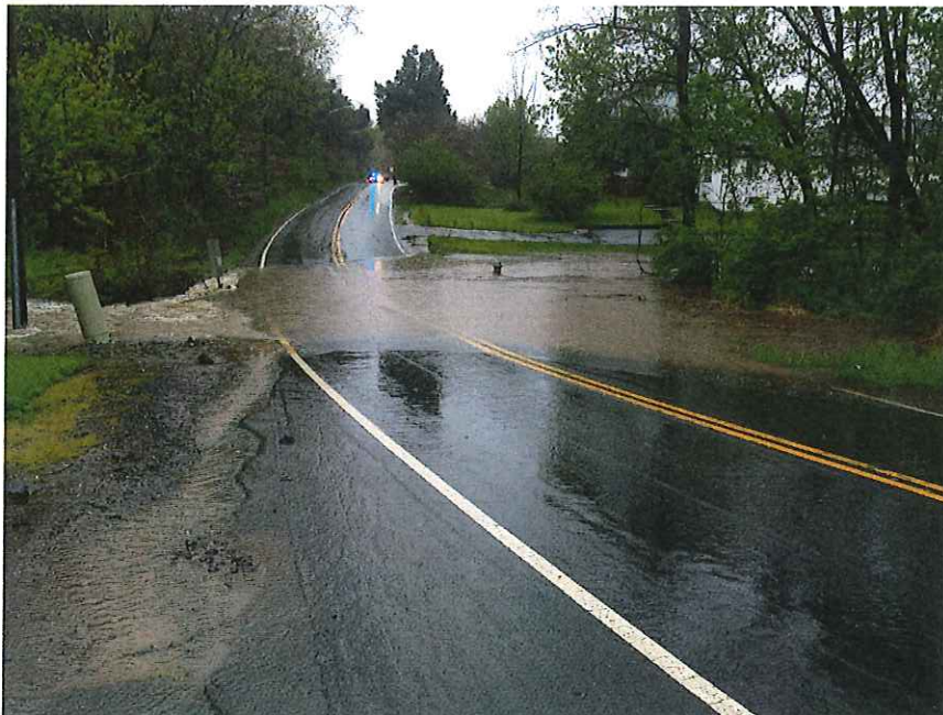
Foothill Type Flooding
